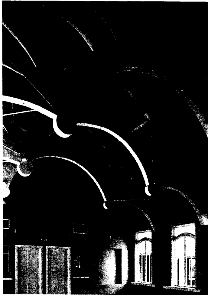
FIG. 10. Completed Truss (Photo © Mark Darley/Esto)
