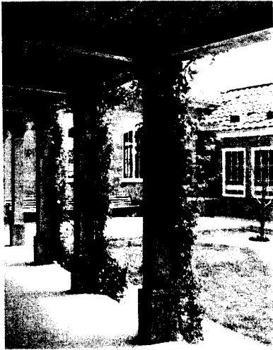
FIG. 1. Homeless Shelter, San Jose, Calif., 1989; Passage and Court with Exposed Timber Framing, Precast Concrete Columns, and Concrete Block Walls: Design by R. Gary Black and Chris Alexander of the C.E.S. (Photo © Mark Darley/Esto)
